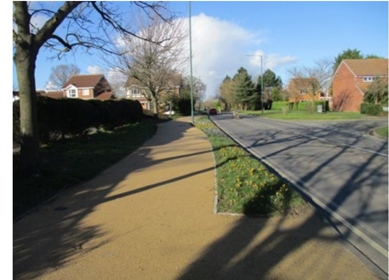
Fig. 16 The 2.5m wide porous shared surface, with bulb planting helping provide a source of pollen for early pollinators
