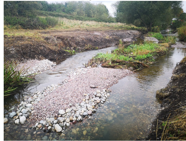
Fig. 11 Wetland works at Kingshurst Brook
